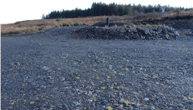
Plate 15: T6, looking SE.
