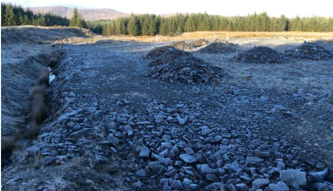
Plate 42: Hardstand at T15, looking NW.
