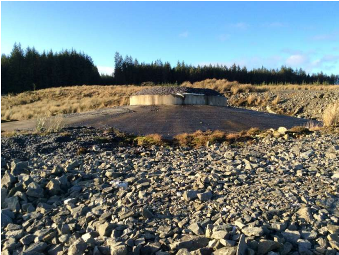
Plate 1: Concrete base at T1, looking NW.
