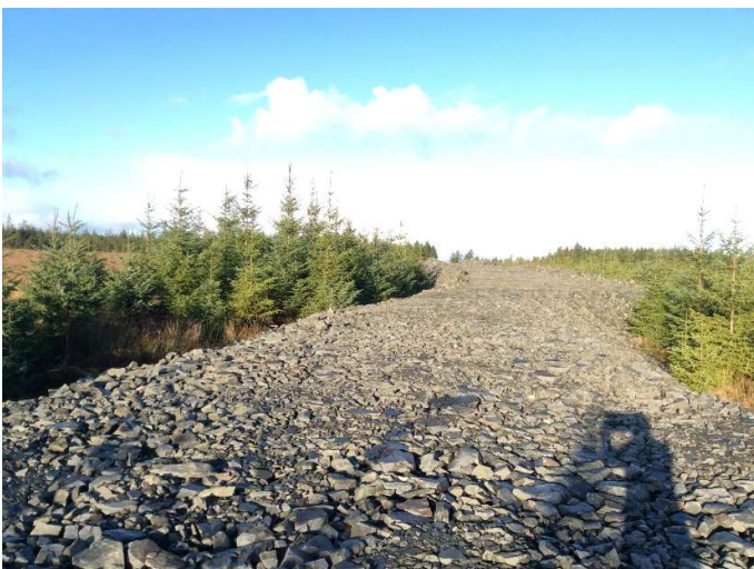
Plate 21: Existing road to T7, looking N.
