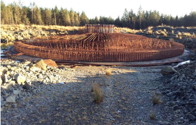
Plate 4: Existing steel for turbine foundation at T2.
