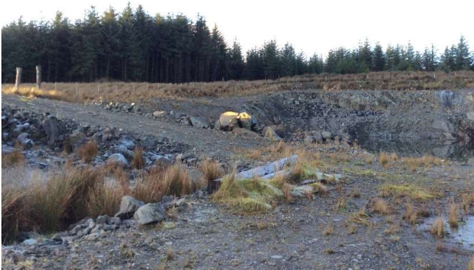
Plate 49: Partially constructed peat cell to be completed N of T18, looking NW.
