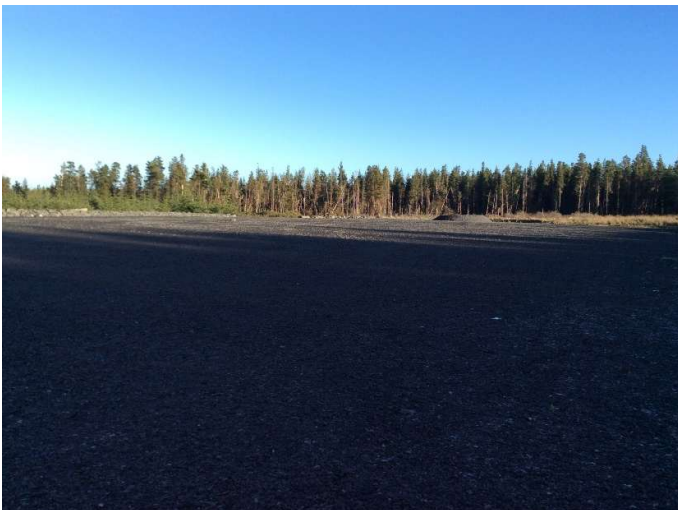
Plate 33: Hardstand and turbine base at T11, looking ENE.
