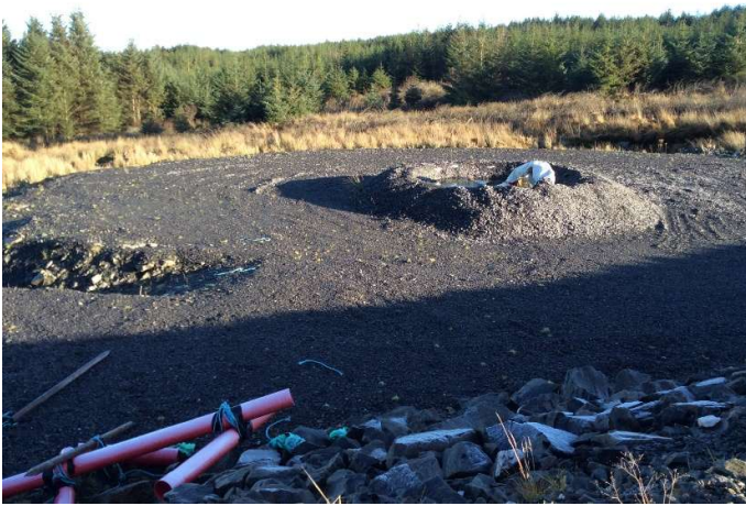
Plate 35: T12 base, looking NE.
