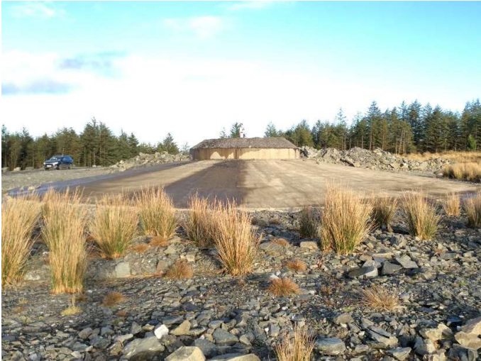
Plate 13: Existing concrete base at T5, looking NE.
