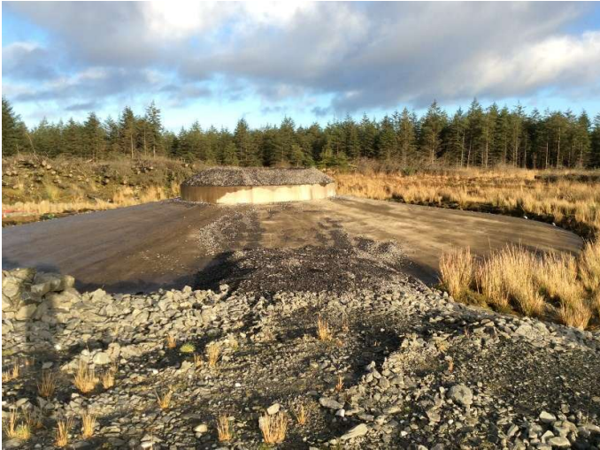
Plate 10: Existing concrete base at T4, looking NE.
